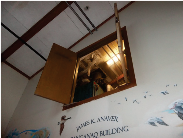
Mechanical Room Access
