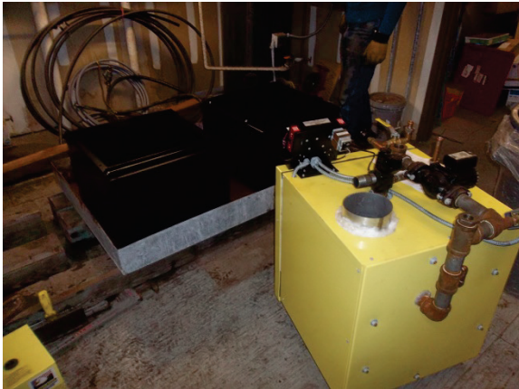
New Boiler Installation
